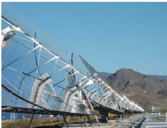
parabolic trough collector
