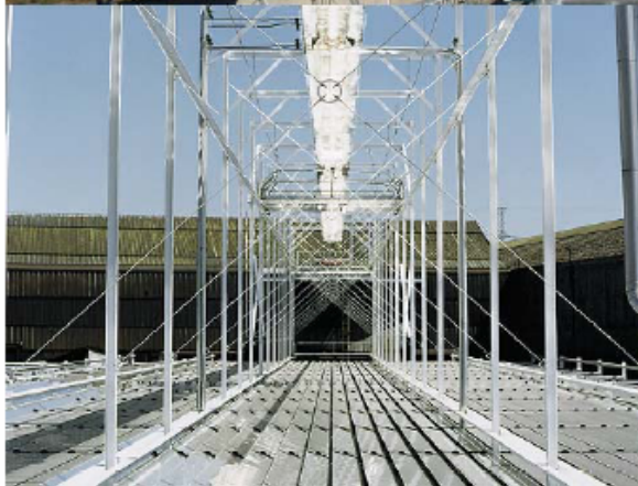
linear Fresnel collector
